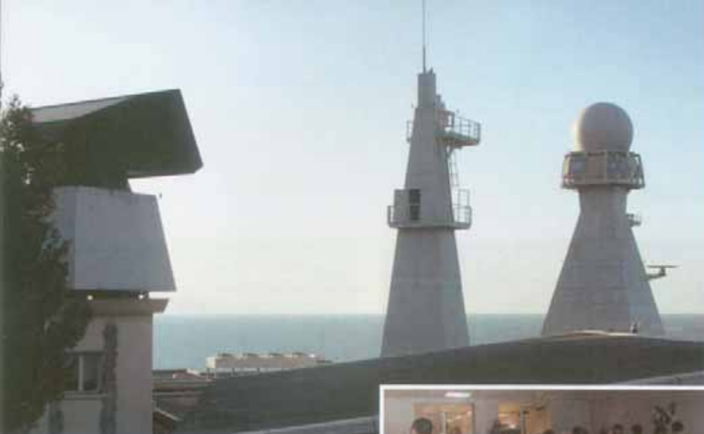
Fig. 6: This is the topside replica of the HORIZON masts, with the CIC replica (see inset) and centres for testing individual elements like PAAMS or EMPAR underneath: the Shore Integration Facility (SIF) in Toulon-Saint Mandrier, to test the software and integrate it with the hardware into the combat system before putting it on the platform, saving cost and time.
